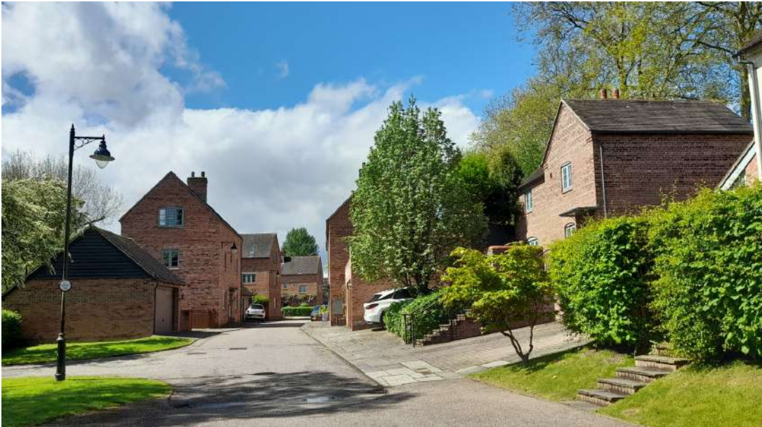
Figure 18: Building set in line with existing buildings with brick boundary wall to edge of street. Using a good brick match for adjacent historic building, sympathetic roof pitch, chimney stacks, sash windows, six panel door with door case, boundary wall and iron gate.
