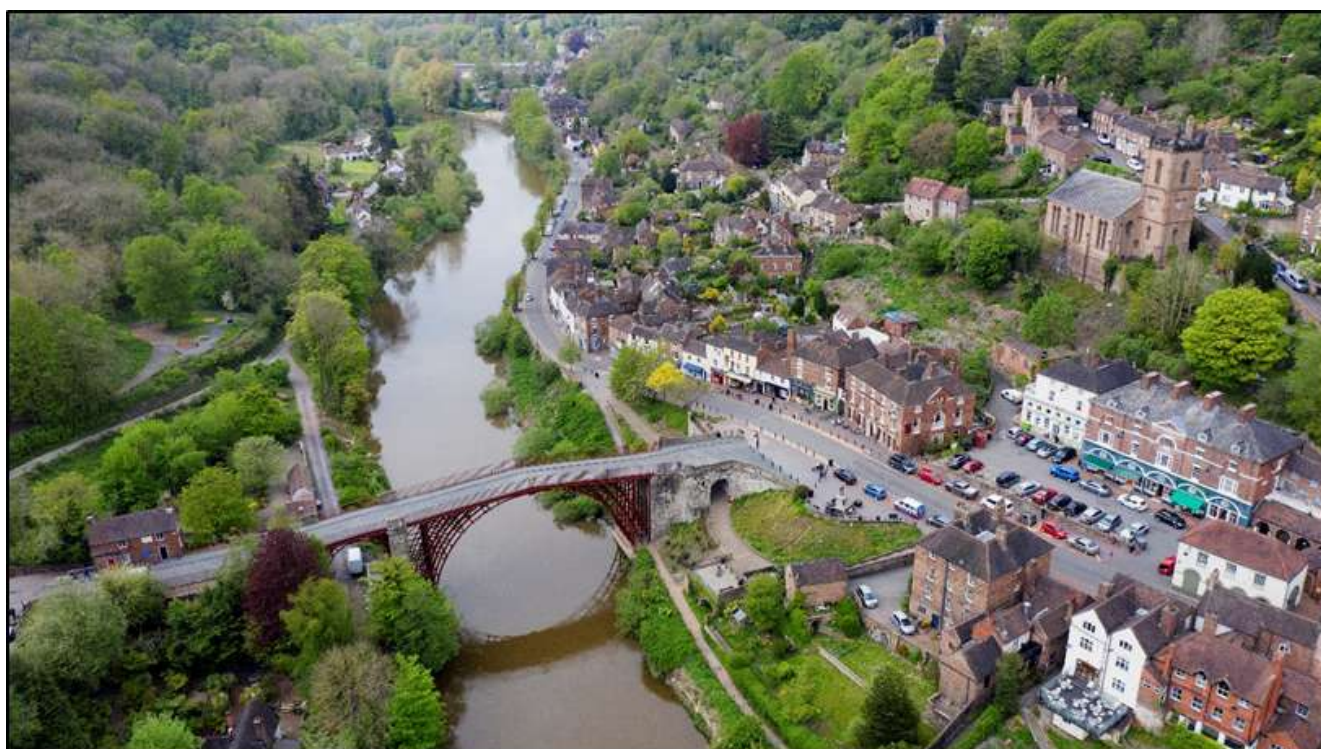
Figure 4: Aerial View of Ironbridge
