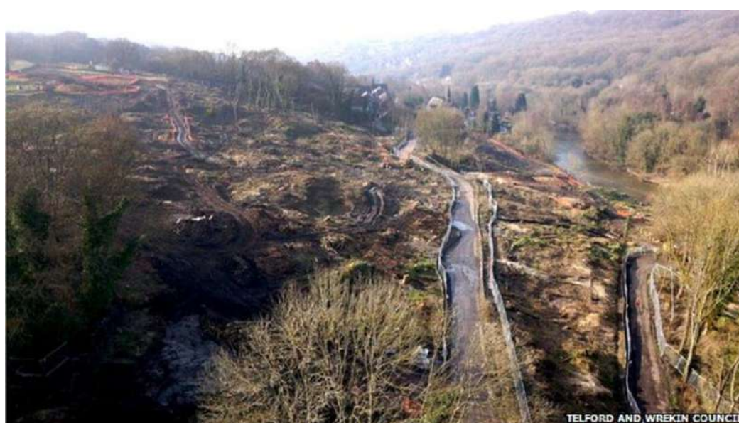
Figure 15: Work to address land instability between Jackfield Tile Museum and Boat Inn
