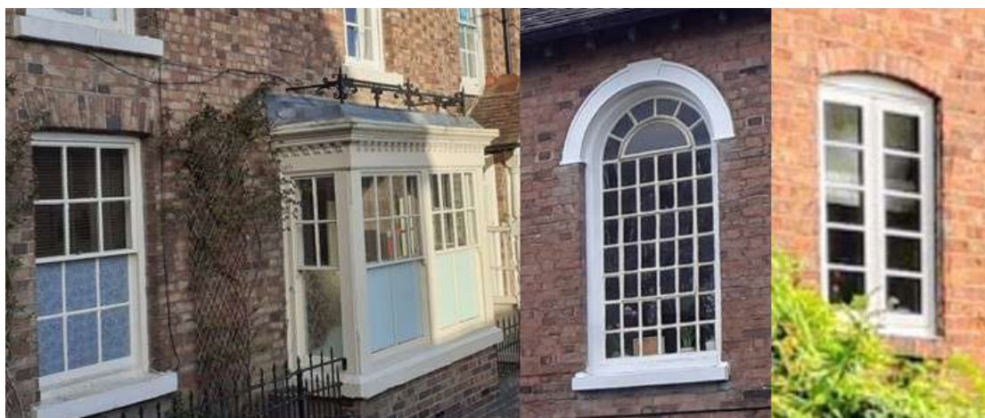
Figure 26: Historic windows in the IGWHS should be retained and used to guide the design and materials of new: vertical sliding sashes, cast iron window, ladder style casement
