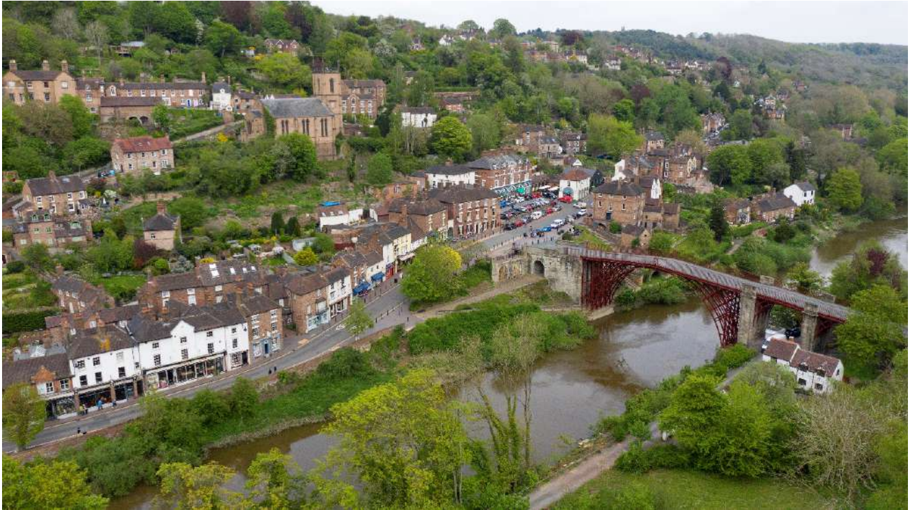
Figure 5: Aerial View of Ironbridge
